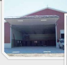
**Easy Installation.** We assemble and jig weld the 4-inch deep tubular frame at our shop and then lift it, as one piece, into place at your building. Insulation and accessories can be easily added on site to customize the door to your exact needs. **Fast Operation.** Midland Hydraulic Doors will open 25 percent faster with just the push of a button. The fast cycle time and power of a hydraulic door will help you be more productive.
